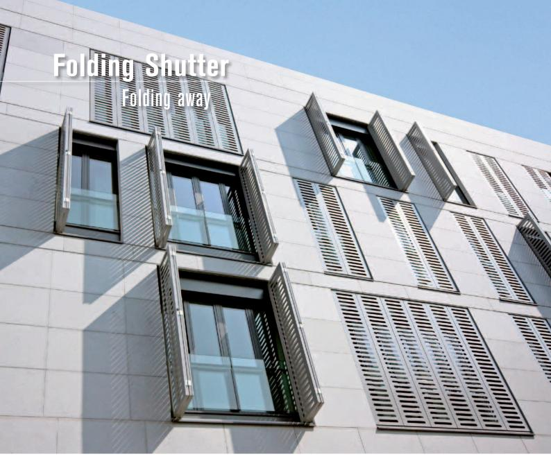
For many years Hunter Douglas has built folding shutters in projects as manual or motorized sun control solution. Folding shutters give a strong dynamic effect to a building by radically changing the facade from a closed, monolithic volume to an open, transparant envelope. The panels fold away from the façade, literally creating an extra dimension that makes this transformation even more dramatic.
