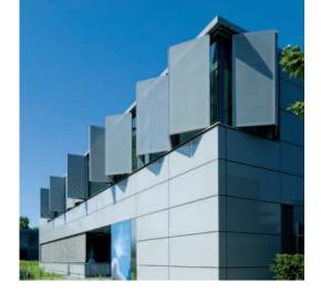
HunterDouglas® Folding Shutters are typically built in aluminium with either fixed louvre fins or a perforated aluminium sheet panel, but can also be provided with any custom material. This allows a complete integration in the surrounding façade. Shutter width can vary from 530 to 900 mm and shutter height can be up to 3600 mm, depending on situation and wind load.
